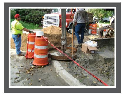
You have challenges, we have solutions! The PENGO Pan Auger is a shallow auger that was designed to be used in retrieving large rocks and boulders out of a hole. A 4" hard-faced flight guard protects the rocks from falling off the edge. A pilot bit and/or special tooth options may be added for a combination of drilling and retrieving.
